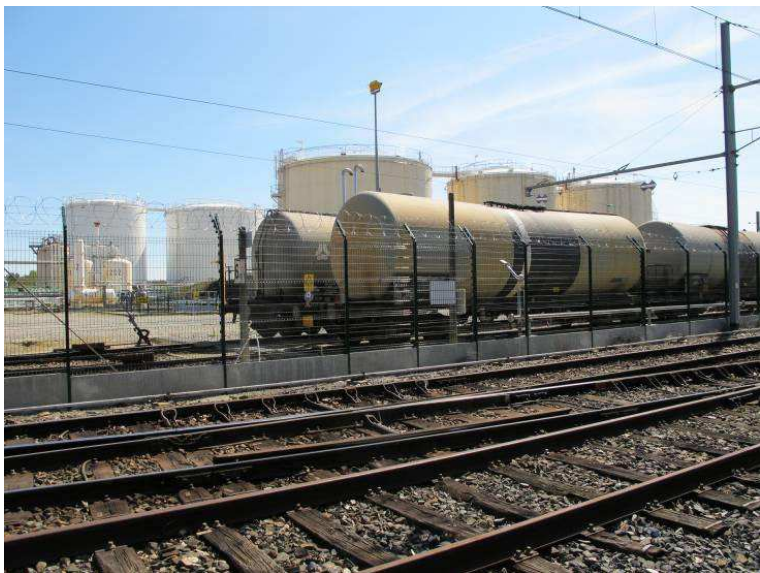
Figure 11: Site TOTAL Raffinage Marketing de Lespinasse (Source : Systra)
