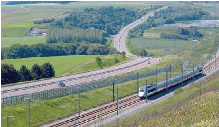
Figure 41: Jumelage LGV EE et autoroute A4 (Source : Egis Rail)
